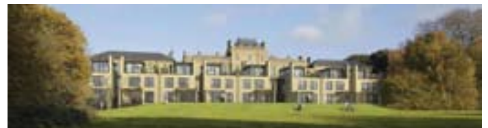
Berkeley's Atkinson Morley scheme in Wimbledon
