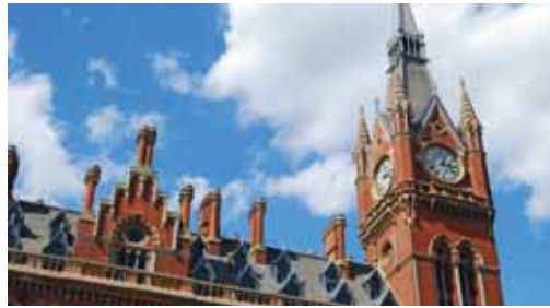
The refurbished St Pancras Hotel
