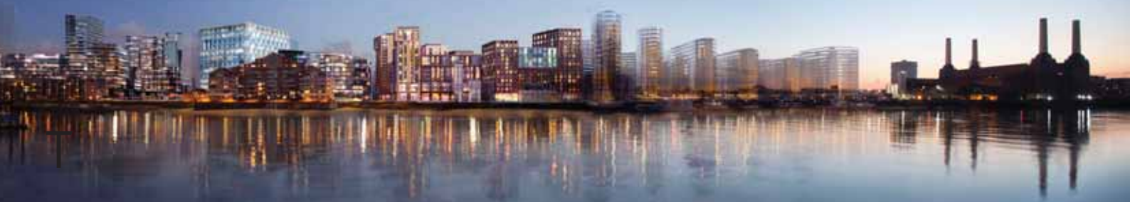
View of proposed development near Battersea Power Station, centre is Embassy Gardens designed by AHMM
