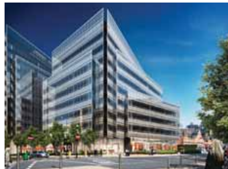
Hammersmith Grove wouldn't have happened with CIL
