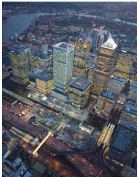
Crossrail at Canary Wharf
