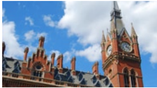
The refurbished St Pancras Hotel
