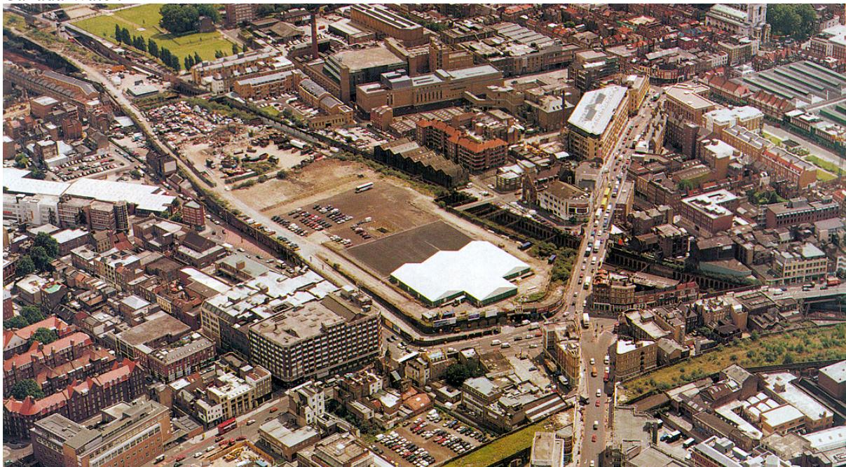
Goods Yard prior to works
