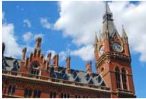
The refurbished St Pancras Hotel
